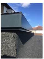
Centralise the inside of the roof with the internal upstand, this will allow the plasterboard to fit neatly into the plasterboard pocket.
