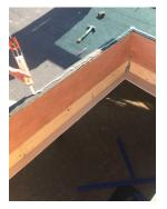
Make sure the roof has an overhang all round, to allow water to discharge.
